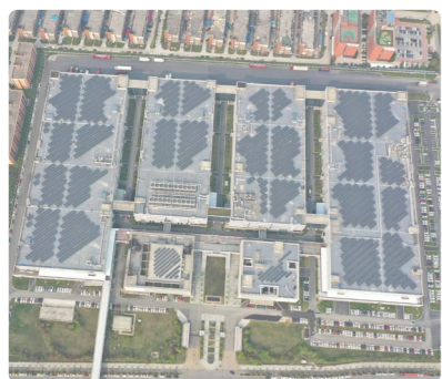
Photovoltaic Project of Nanchang No. 1 Manufacturing Center
