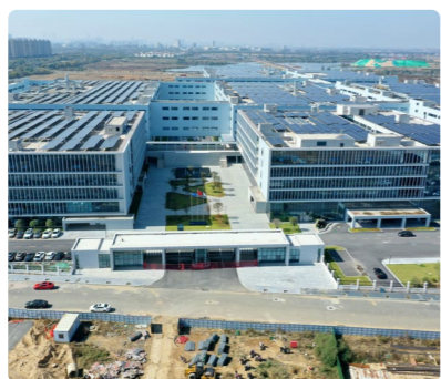
Photovoltaic Project of Wuxi R&D Center
